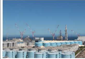
TEPCO's Fukushima Daiichi Nuclear Power Station
